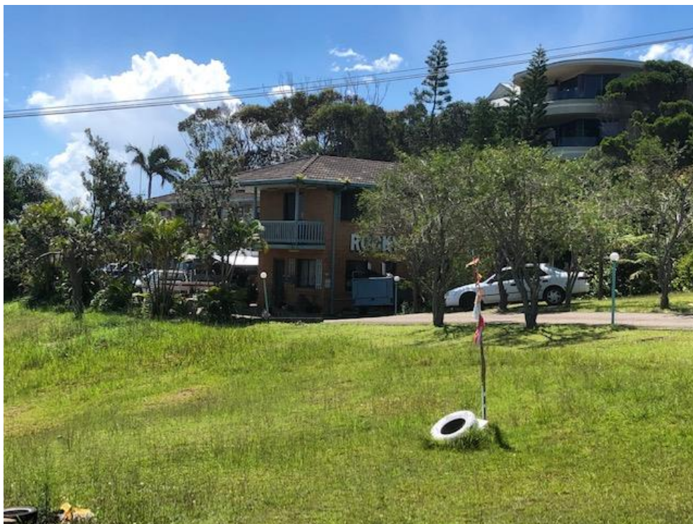
Existing motel building in the northern portion of the subject site
